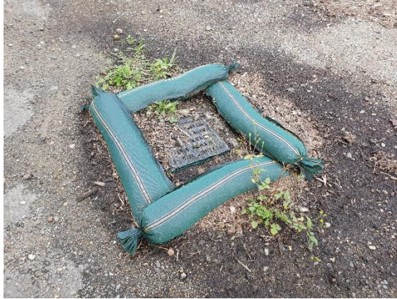
Photograph 14: Example of blocked square drain.
