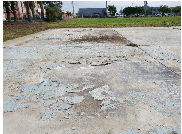
Photograph 12: Example of weathered thick textured paint on southern portion of concrete slab. View east. (April 2020)
