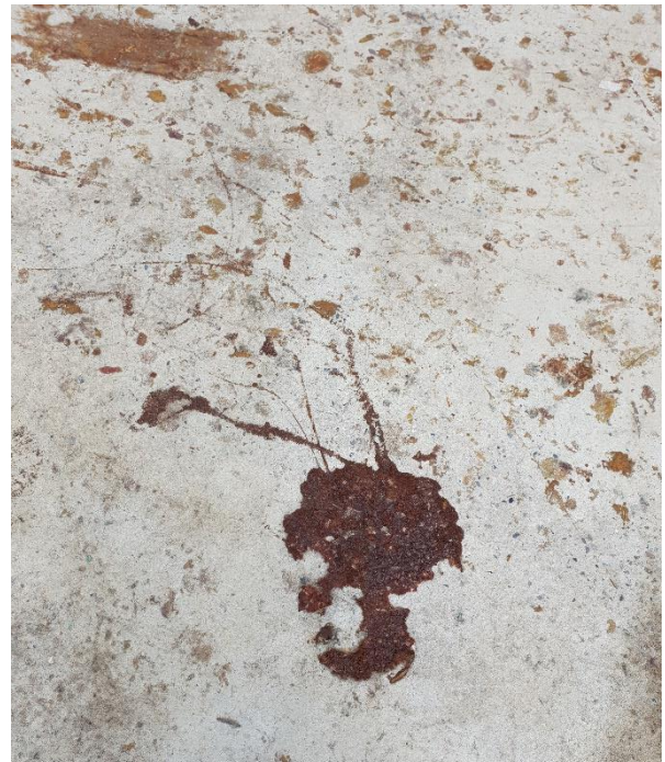
Photograph 6: Iron/rust staining observed in north eastern portion of slab. (April 2020)
