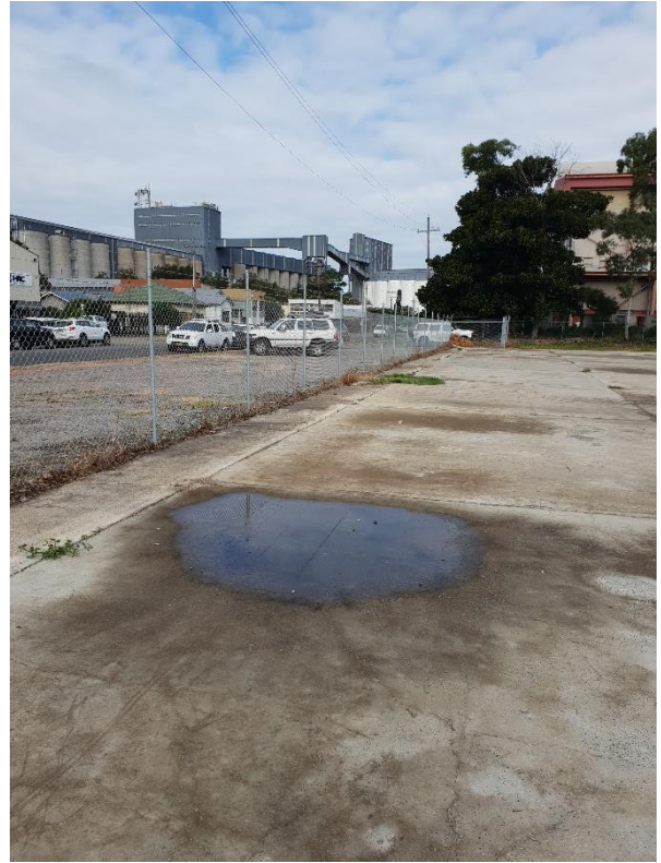
Photograph 8: Surface water pooling on slab following rain event. View south. (April 2020)
